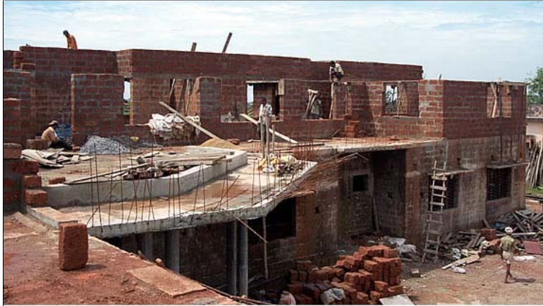
(PIC)State of construction as of Oct 2007
